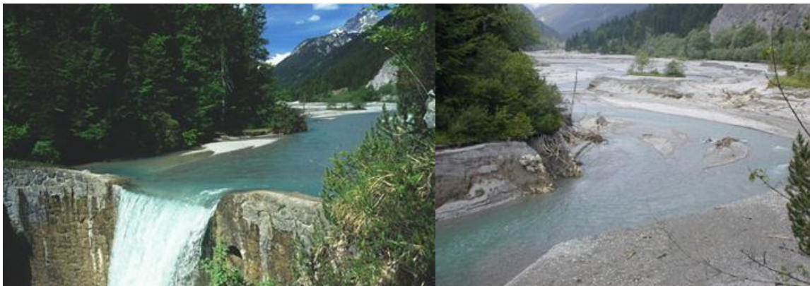
Figure: Sediment re-activation at a small highland river by dam removal, at a tributary to the river Lech in Tyrol, Austria (situation before/after dam removal – Photos: Ch.Moritz).
